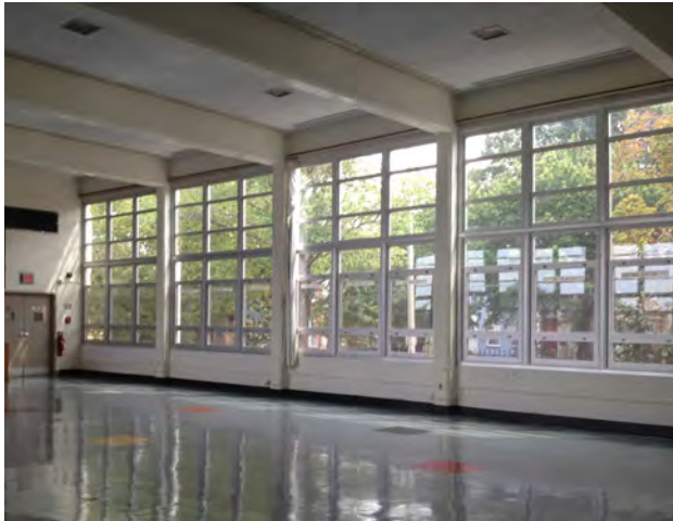
Figure 5.17: Excellent access to daylight and exterior views in the auditorium of Prospect Learning Center in Washington, DC
